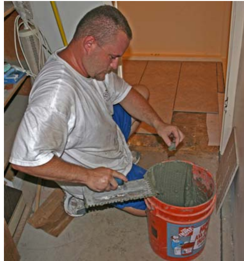
Brandon Baughn laying tile ↑
