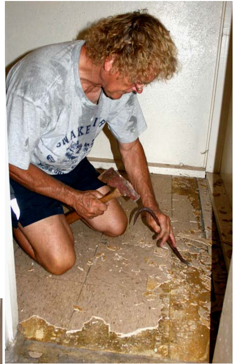
Wayne chipping up tile ↑
