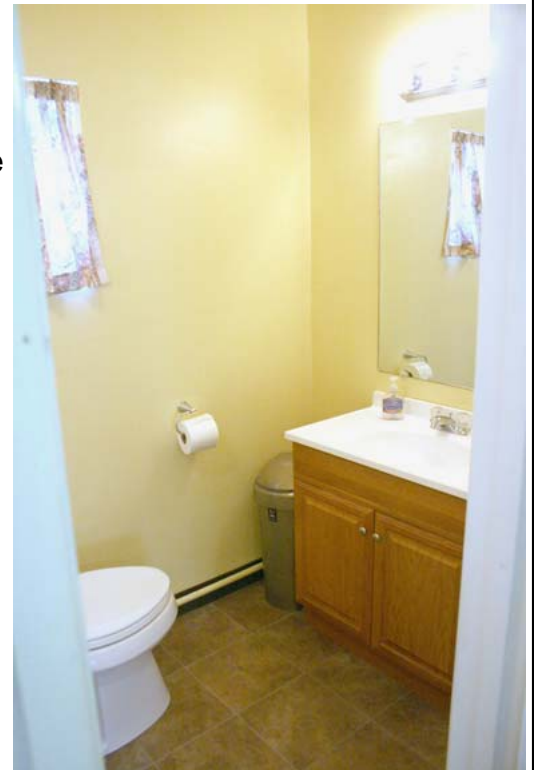
New paint, toilet, tile, vanity, light bar, and towel dispenser.
